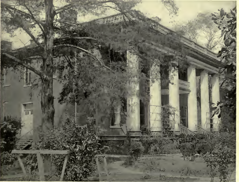
FIG. 9.—HOUSE IN TUSCALOOSA, DATING ABOUT 1845. The front is stucco on brick, painted to imitate pink marble.
